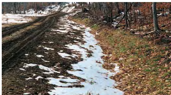
Revegetated road ditches carry water without eroding.
