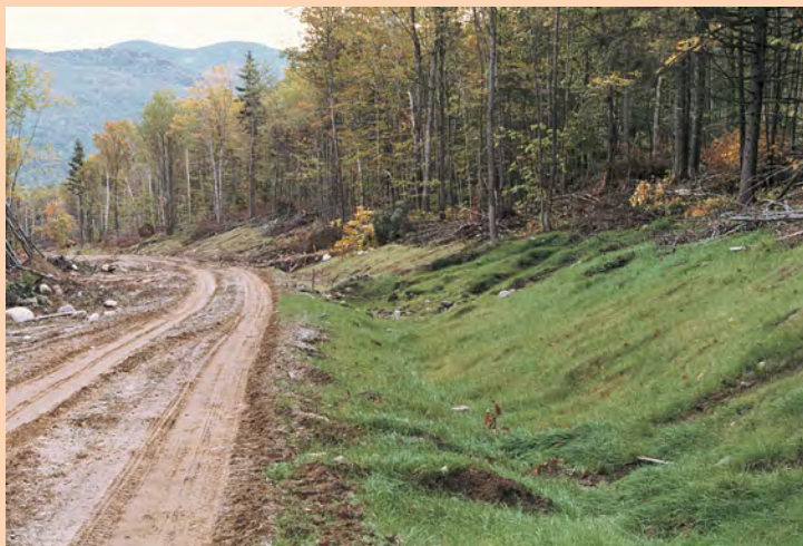
Hay mulch holds exposed soil while grass becomes established.
